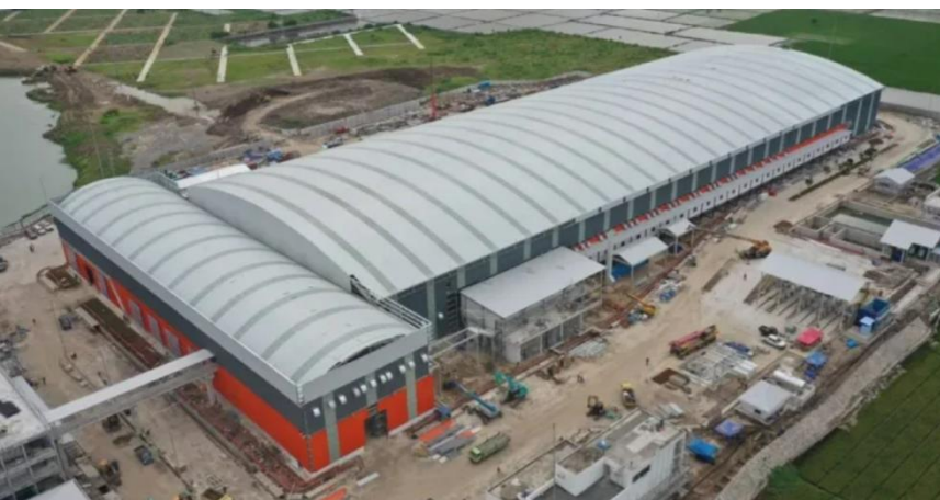
Gambar 2.11 RDF Plant Rorotan
